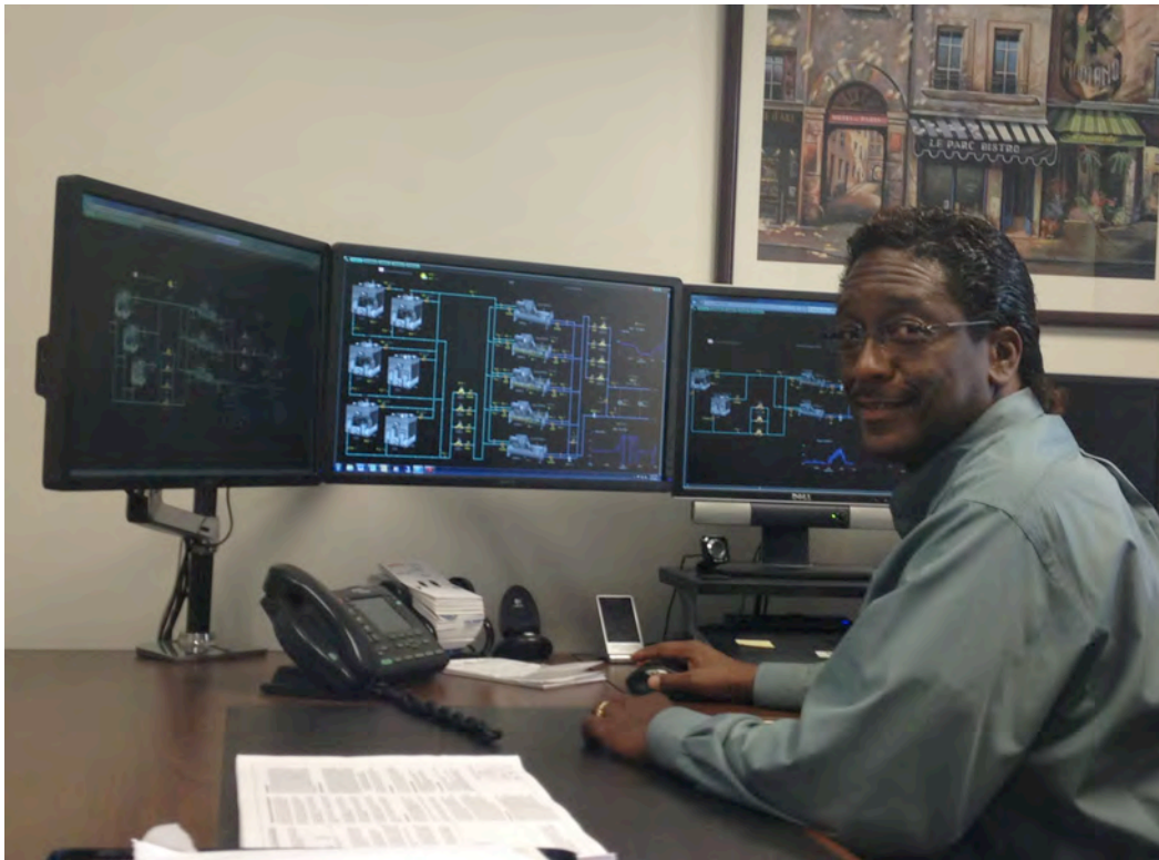
Figure 2.14. ALC Building Automation System controls all HVAC systems college-wide from a central point. Robert Hickman, Operations Manager, Energy Efficiency leads the effort, and several other staff members can operate the system.
